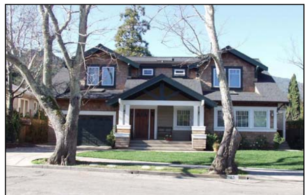
Figure 10 – New second-story addition is compatible with the existing residence.
