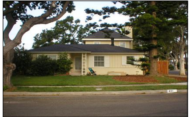
Figure 20 – Second-floor addition replicates the existing ground floor design and materials.
