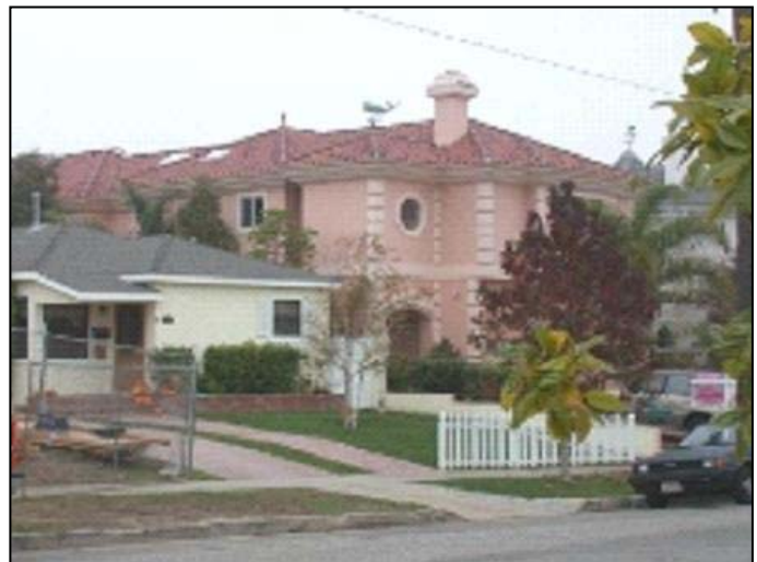
Figure 7 – Incompatible mass and scale of adjacent residence shown on the right.
