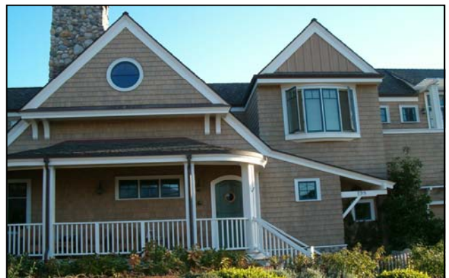
Figure 21 – High quality, authentic materials are incorporated into the design to enhance the architectural style.
