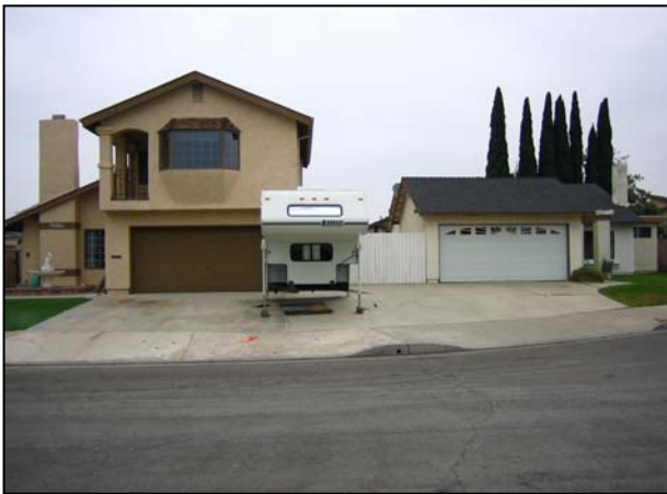
Figure 11 – Second-story addition is located within the side yard encroachment plane.
