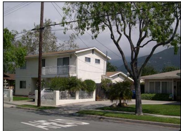
Figure 9 – New addition size and scale is incompatible with the existing residence.
