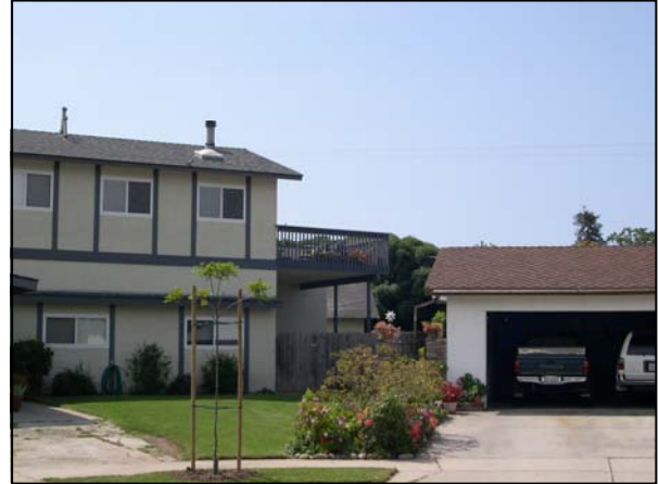
Figure 22 – Second floor deck creates privacy issue for adjacent residents.
